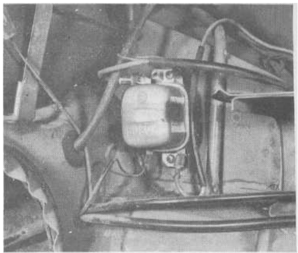
11.1 The regulator is behind the air cleaner in the engine compartment
